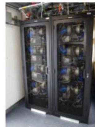
(2) HyPM™-R120 installed within sea container (240 kW<sub>gross</sub>)
